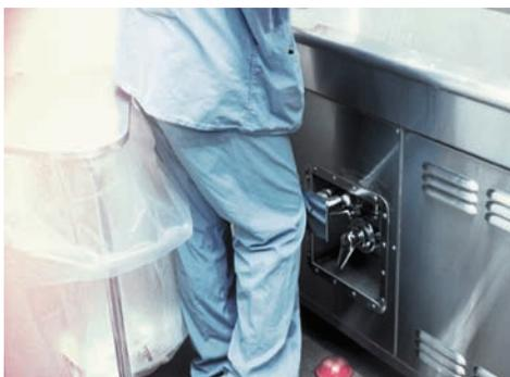
**FIGURE 29-47** Handwashing Sink with Knee Controls. DELMAR/CENGAGE LEARNING
